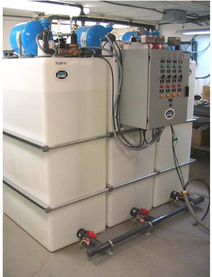
The unit shown is made of three SSPB210WSV100-20 Herculan ConstaBoost Static Storage Systems connected and controlled by a CNT-SJE4PMP-ALT. The system can be expanded as the control will operate 4 of these units. As seen the system stores 600 gallons of water can deliver 66 gpm at 55 psi. The system fill rate is adjustable 0-18 gpm.
